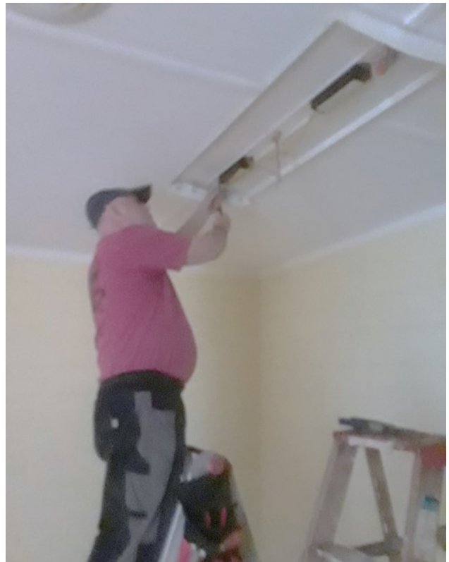
Dan changed out the light fixtures for LED.
