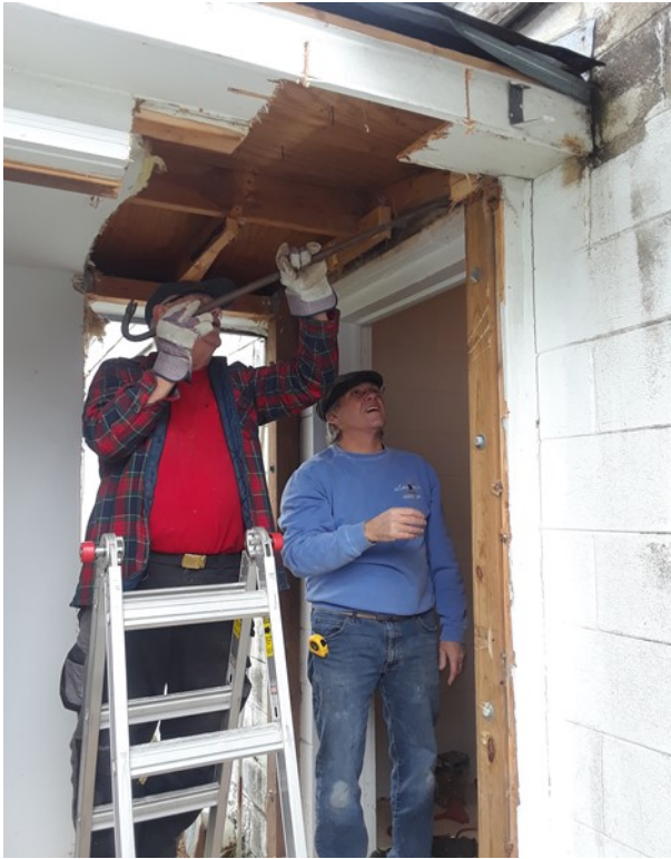
Bob and Dan with help from Jo Ellen removed the connectors so the roofers could rebuild the roof overhang.
